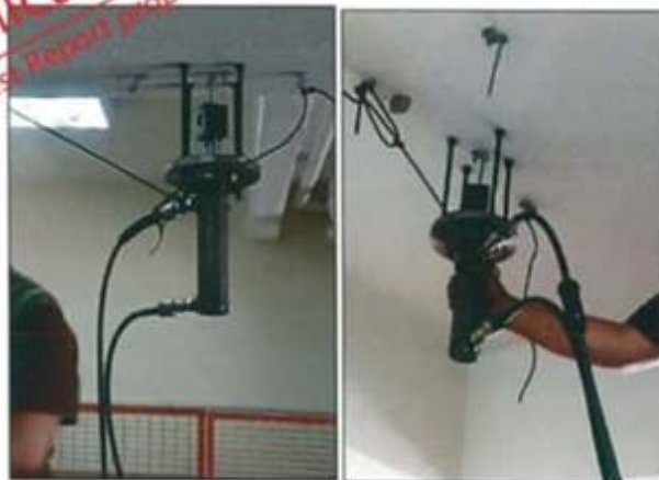
Photo A.5 : Hydraulic hoses installed to complete the pull out fixtures.
