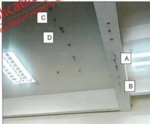
Photo A.2.2 : Identified Fastener Shooting Nail installed at ceiling beam and ceiling slab.
